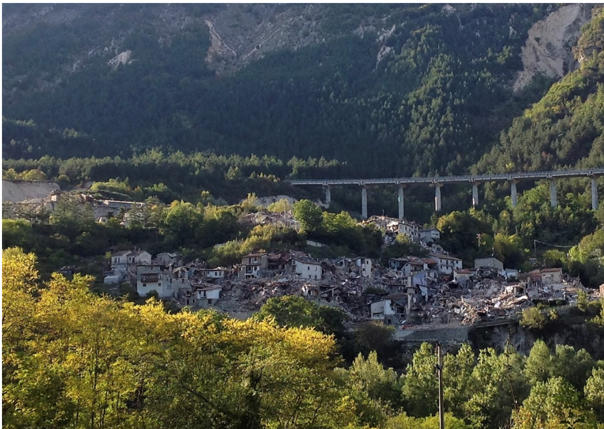
Figure 10: The town of Pescara del Tronto razed by the earthquake.
