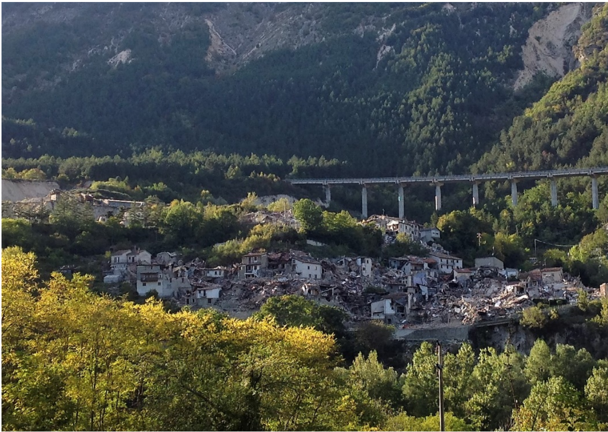
Figure 10: The town of Pescara del Tronto razed by the earthquake of 24 August 2016.
