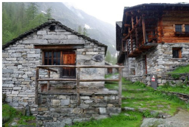
Figure 4. Example of an alpine hut: this is the hut in the Bors valley, the second to be encountered along the geotrail route. Photo by the authors.
