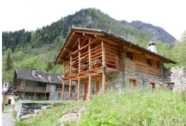
Figure 6. Typical Walser house, an example of vernacular architecture in Alagna Valsesia. Photo by the authors.
